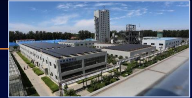
Micro-Grid UEI Demonstration Project in Langfang
